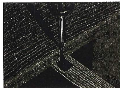
Hidden Fastener Installation to Joist
